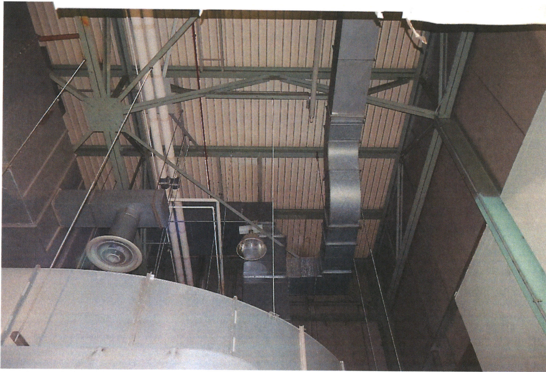
Roof in Retubing Area
