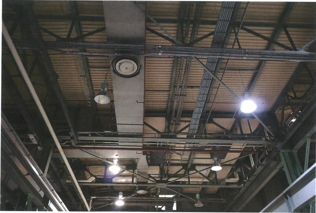
Roof in Retubing Area
