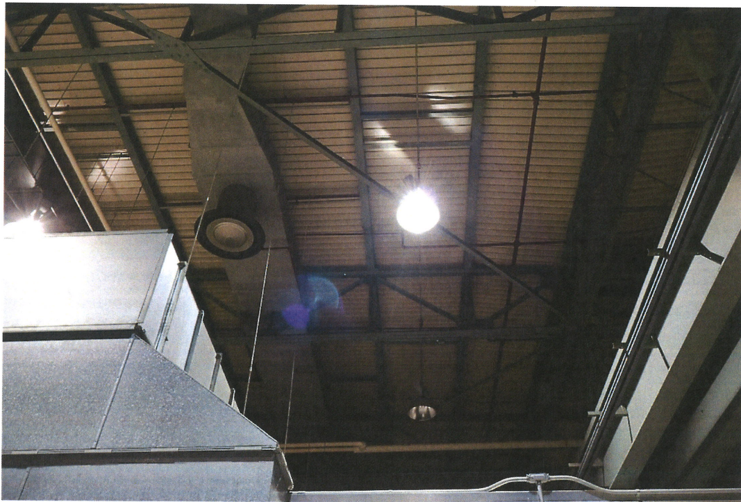
Roof in Retubing Area
