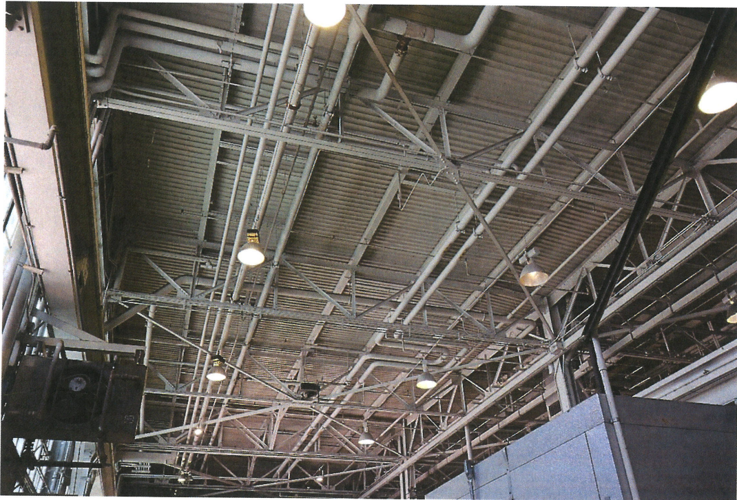
Roof above Shop Area
