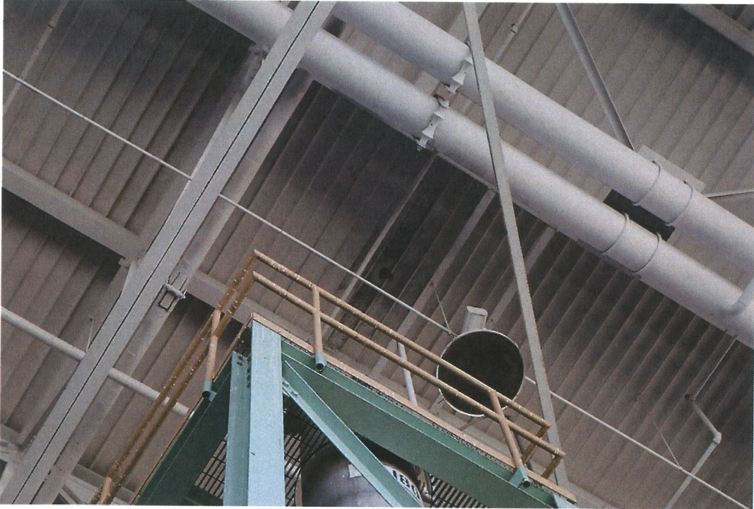
Evidence of some sort of repair near column E12
