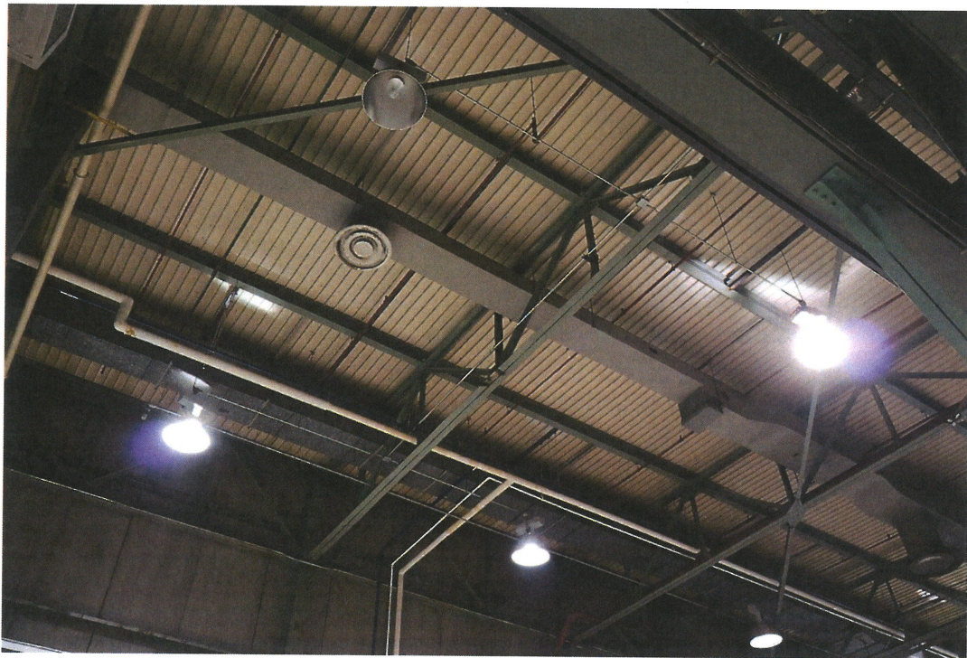
Roof in Retubing Area
