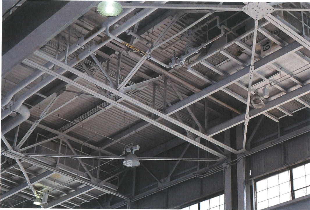
Roof on East side of the Cleaning Area
