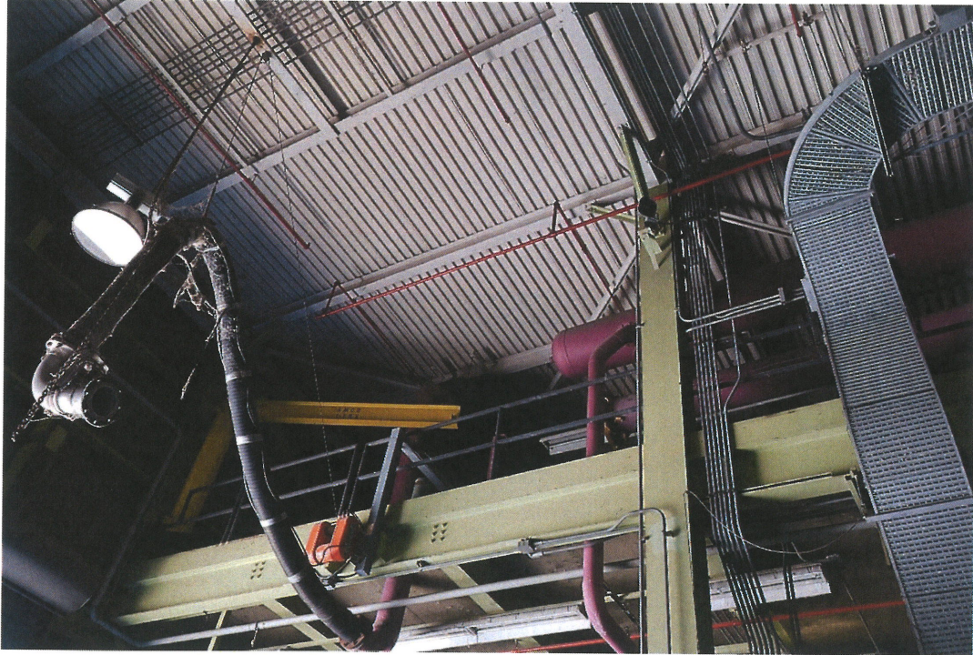
Roof in West building addition
