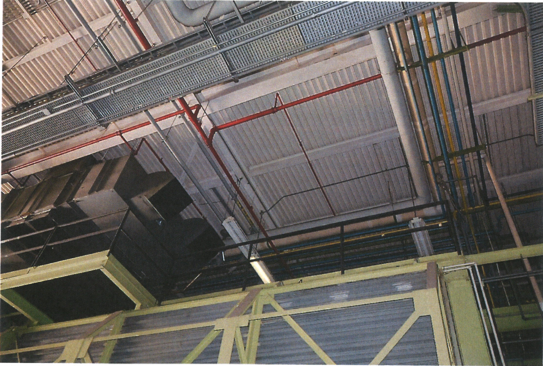
Roof in West building addition
