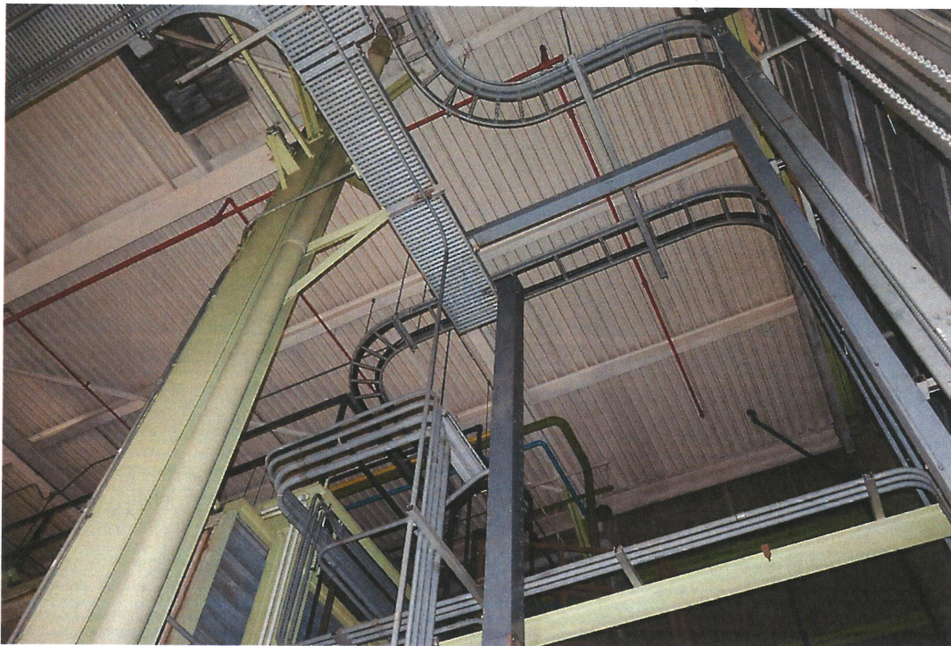
Roof in West building addition
