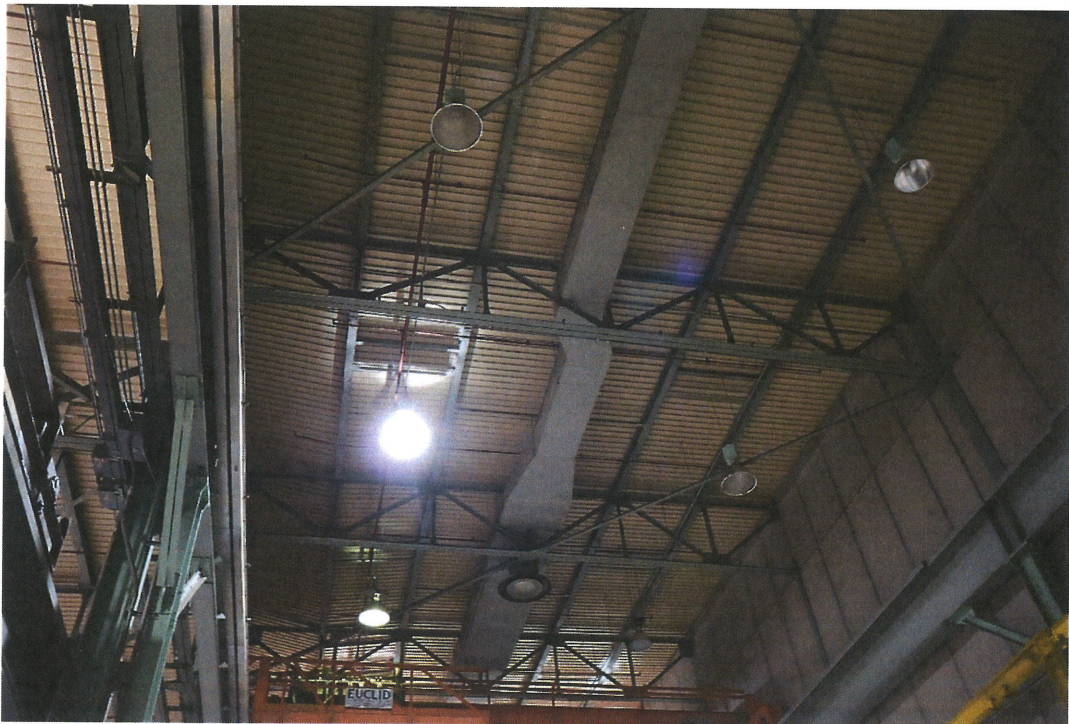
Roof in Retubing Area
