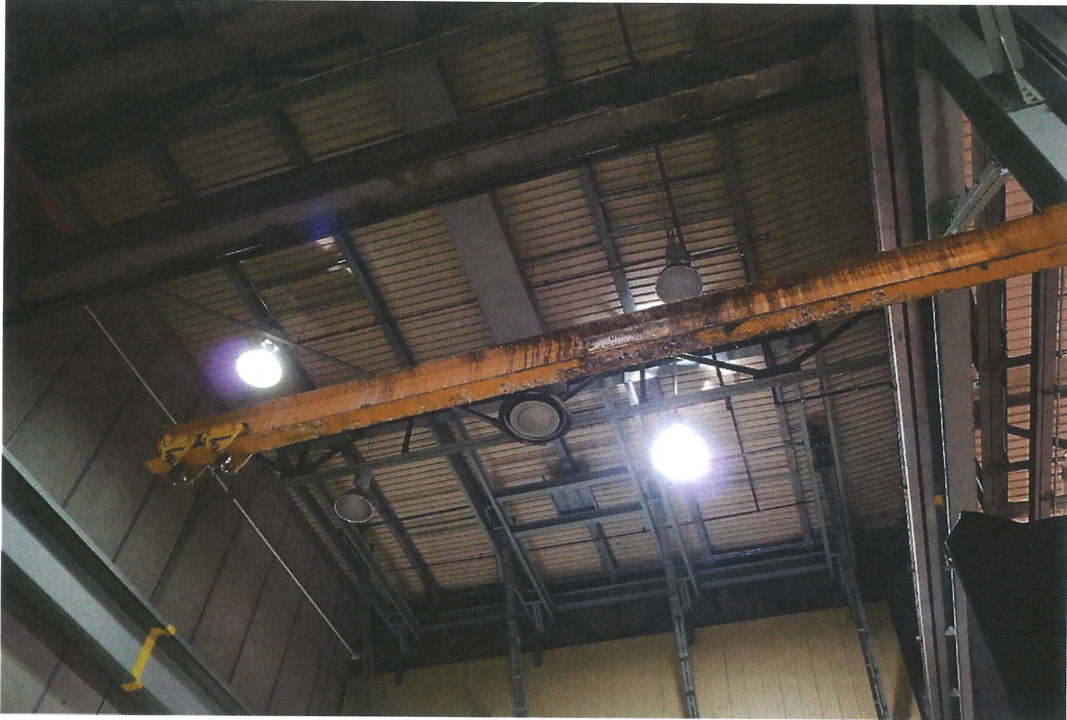
Roof in Retubing Area
