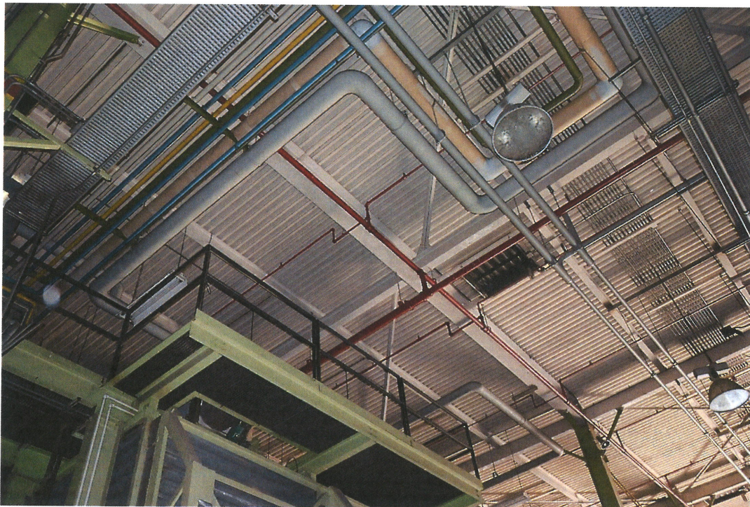
Roof in West building addition
